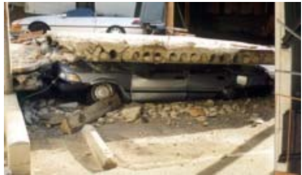
Figure 1. Flattened car under a hollowcore floor unit that has lost its support. [1]
