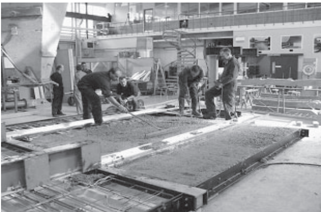
Casting of concrete floor slabs
