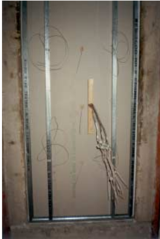
Figure 5-8: Typical thermocouple layout in specimen.
